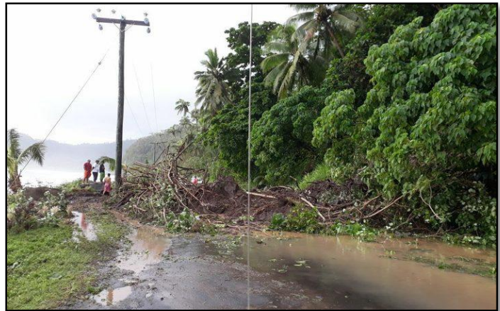
Landslides frequently occurred on the east coast road during heavy rainfalls.
